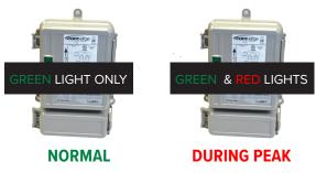
\*IF BREAKER IS TURNED OFF, RCS WILL GO THROUGH A 10-MINUTE START SEQUENCE WHERE LIGHTS ALTERNATE ON/OFF
